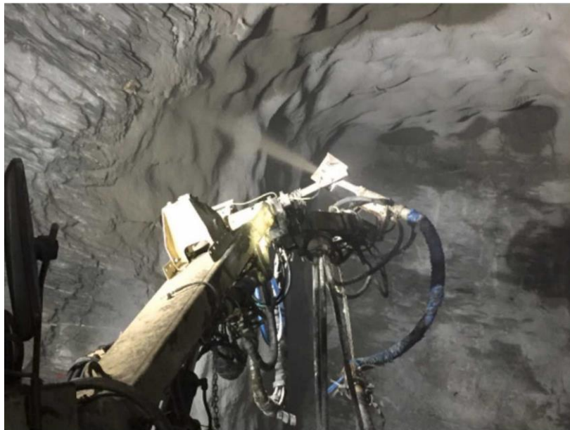
Fig. 3. Application of fibre-reinforced shotcrete - robotic sprayer, Cuiabá underground mine, Brazil, 2021 (23)
