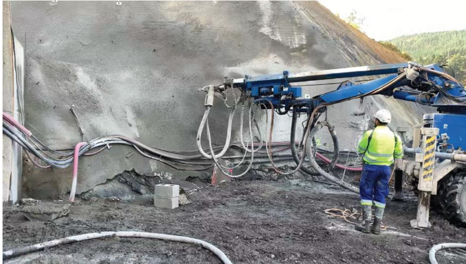
Fig. 4. Strengthening of a tunnel rock slope using shotcrete (High-Velocity Train Sacyr Green, Spain, 2022; source: www.flexofibers.com )
