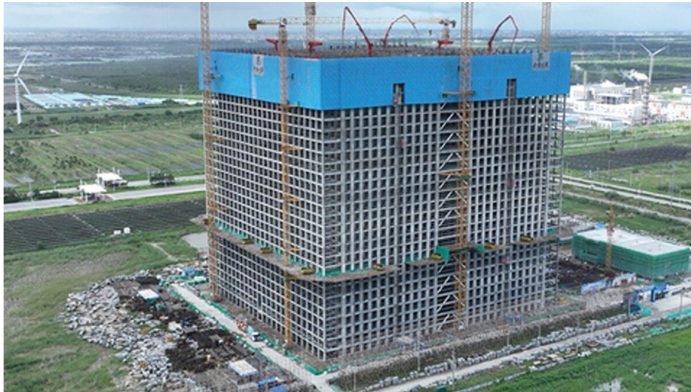
Fig. 3. Energy storage system in, China under construction [Image: Energy Vault, Business Wire]
