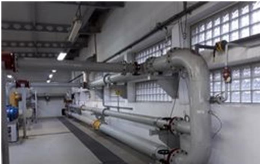
Fig. 4. Outlet pipe arrangement
