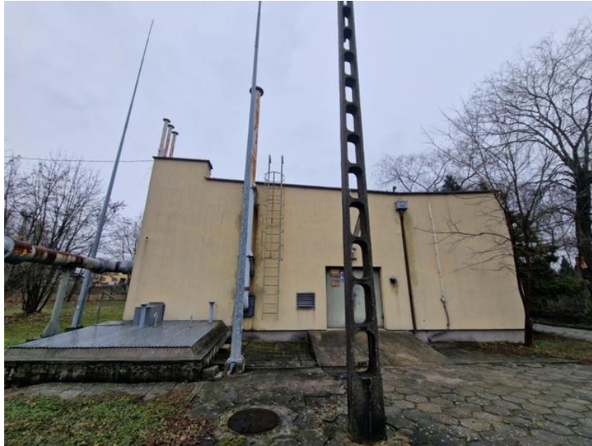
Fig. 1. The building of the methane drainage station
