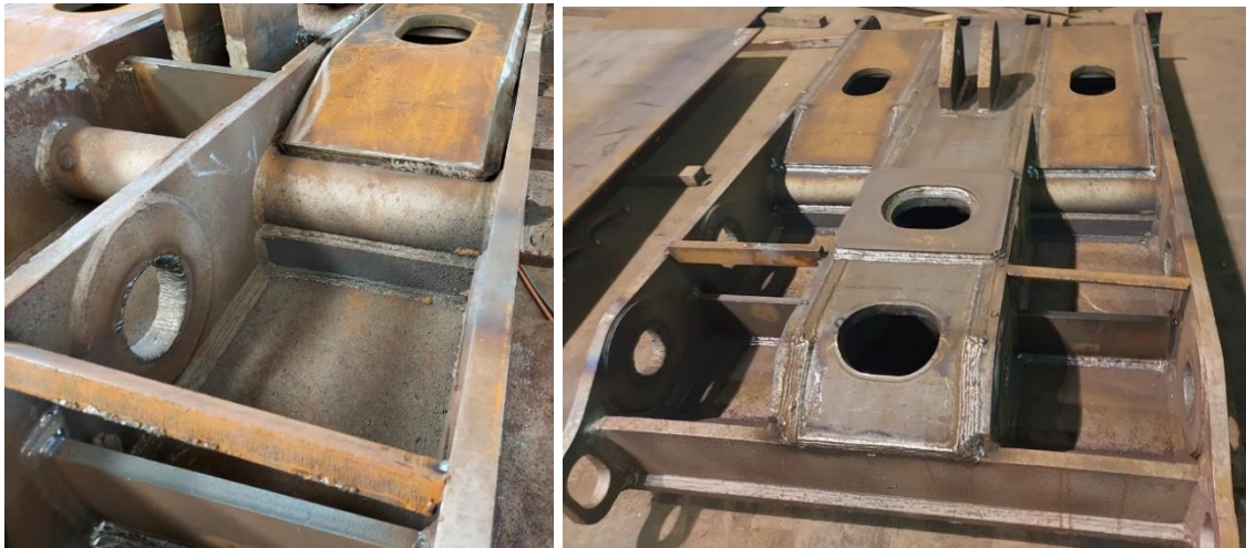
Fig. 6. Welding the details
