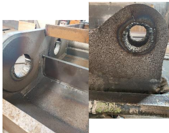
Fig. 5. Welding the openings
