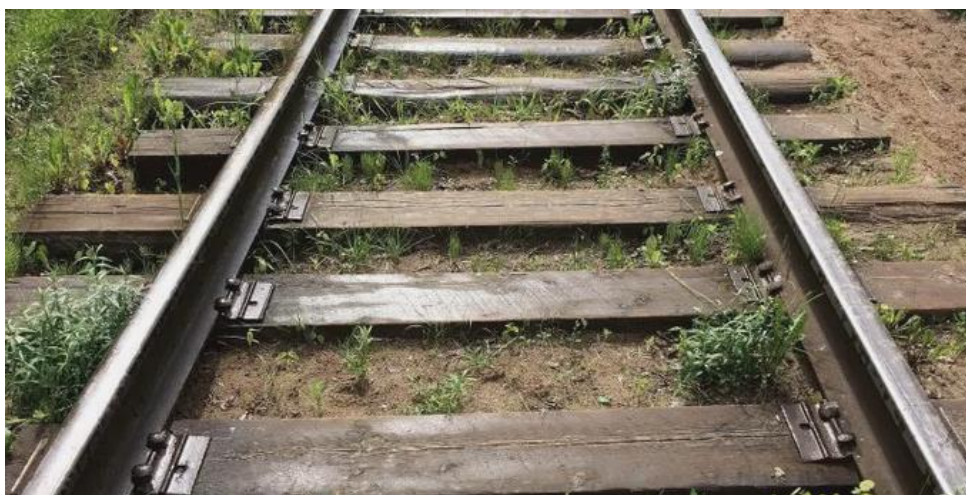
Fig. 1. Impregnated wood in railway sleepers [10]
