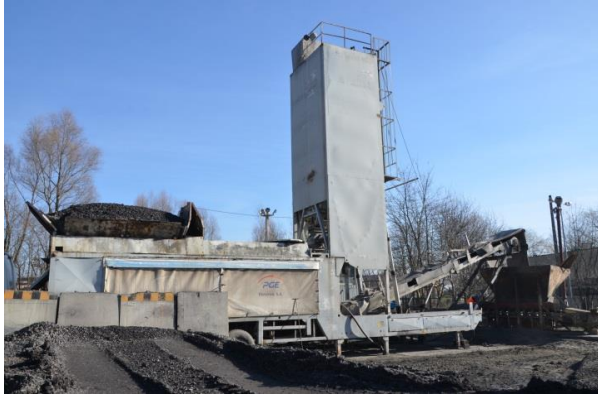
Fig. 9. Installation from the feeding side
