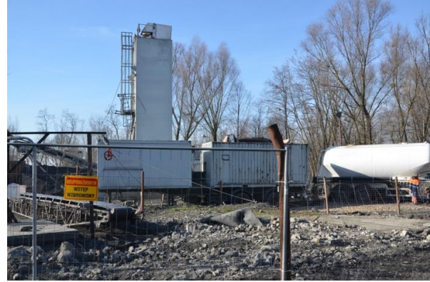
Fig. 10. Installation of discharging to "Jas VI" shaft
