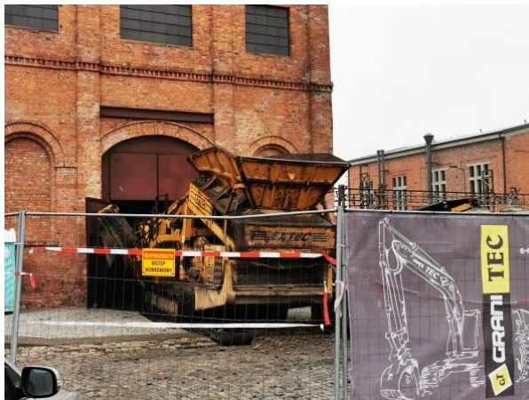
Fig. 5. Position of the screening machine for backfilling
