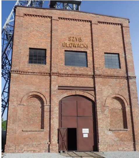
Fig. 3. Building of the „Głowacki” shaft landing
