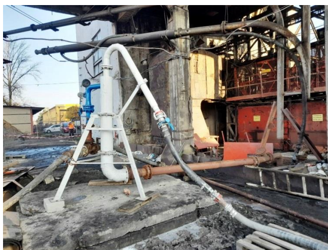
Fig. 8. Feeding the hydraulic binder with the use of a mixer
