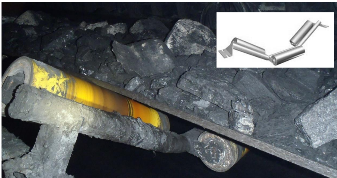
Fig. 1. Roller belt support system in an underground coal mine
